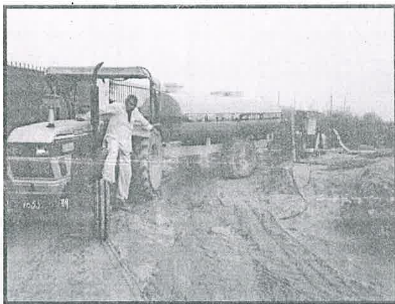
Water Sprinkling at Site.
