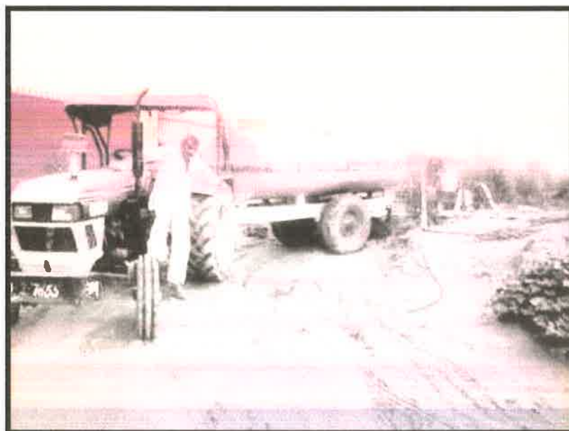
Water Sprinkling at Site.
