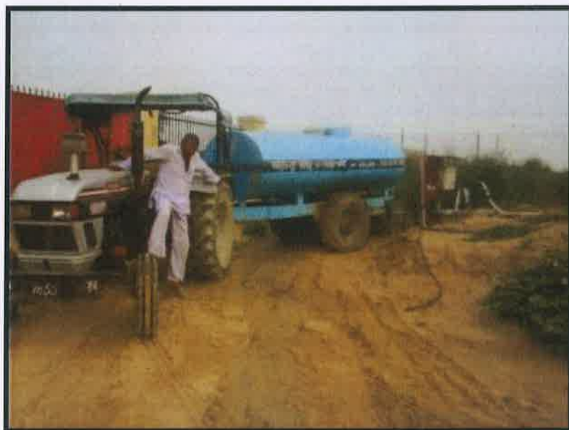
Water Sprinkling at Site.
