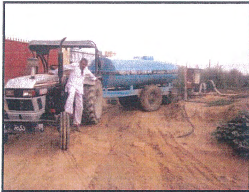
Water Sprinkling at Site.
