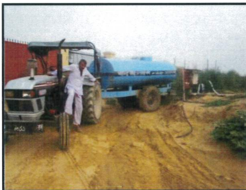
Water Sprinkling at Site.
