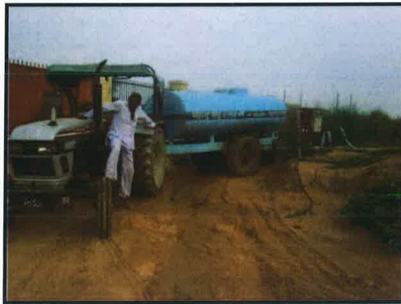
Water Sprinkling at Site.
