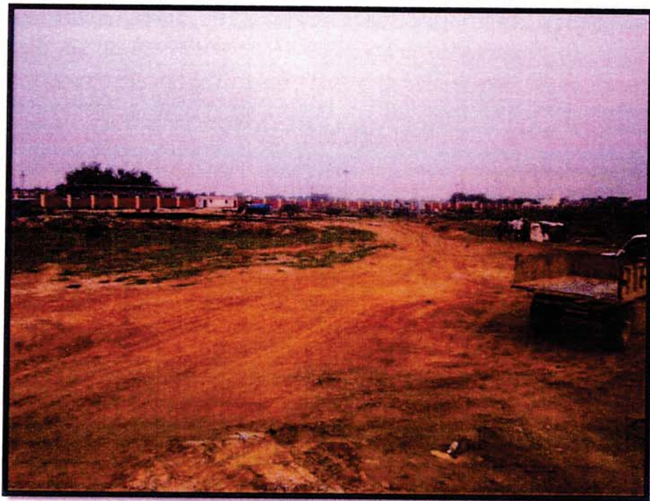
Site Barricade with High wall
