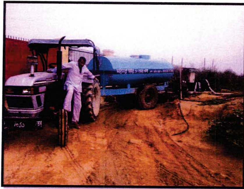
Water Sprinkling at Site.
