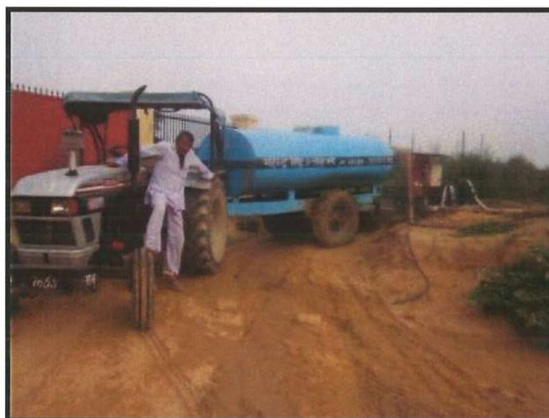
Water Sprinkling at Site.
