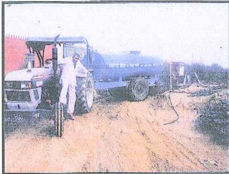
Water Sprinkling at Site.
