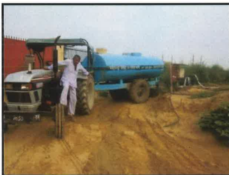
Water Sprinkling at Site.
